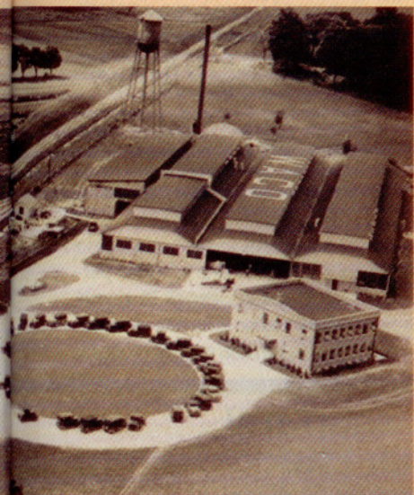
The Waco Aircraft Company plant was located off Peters Pike in Troy, Ohio, in 1929 (above). Aircraft are shown in production at the Waco plant (below).
